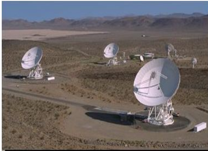
Fig. 2. DSN 3-34m beam waveguide antennas at the NASA tracking station in Goldstone, CA
