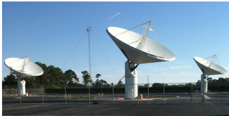
Fig 8. Array of Three 12m Reflector Antennas on a Scalene Lattice
